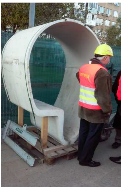
Inlocuire canal colector soseaua Mihai Bravu
